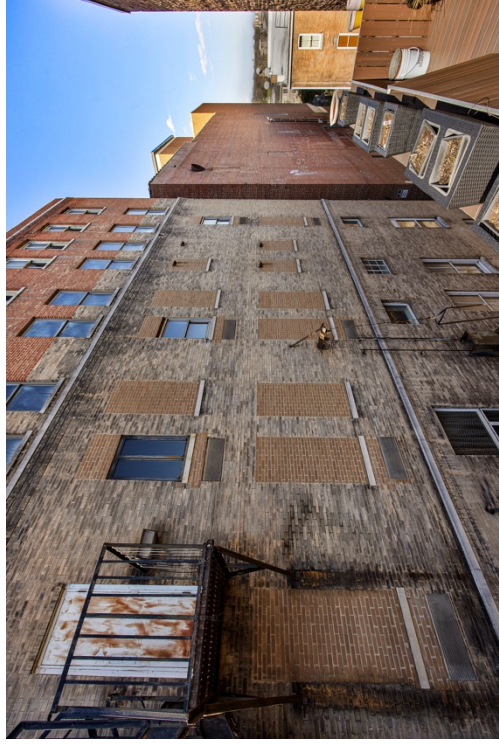
Exterior of 612 S Gay Street
